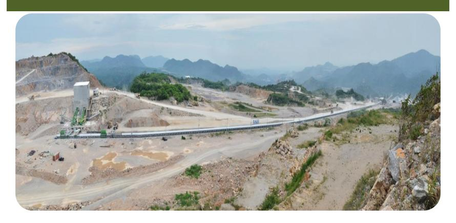
Linked quarry to production facility via conveyor belt saving 3.03m litres of diesel per year, and produce 1.07m kWh of electricity.
