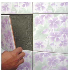
Ceramic tile repairing
