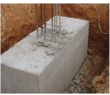
Suitable for Post work, Beam and Foundation Post at compressive strength 350 KSC (or 320 KSC Cube)
