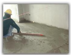
Suitable for Ground Leveling at compressive strength 180 KSC cylinder (or 210 KSC Cube)
